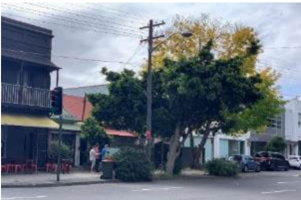
Figure 26. 88, 86, 84, 82, 80 and 44-78 Rosehill Street, Redfern
