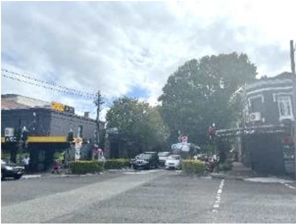
Figure 10. 132 and 134-136 Buckland Street, Alexandria
